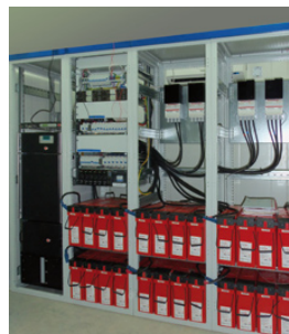
Fuel Cell, Electrolyser, Battery Bank and Power Electronics
